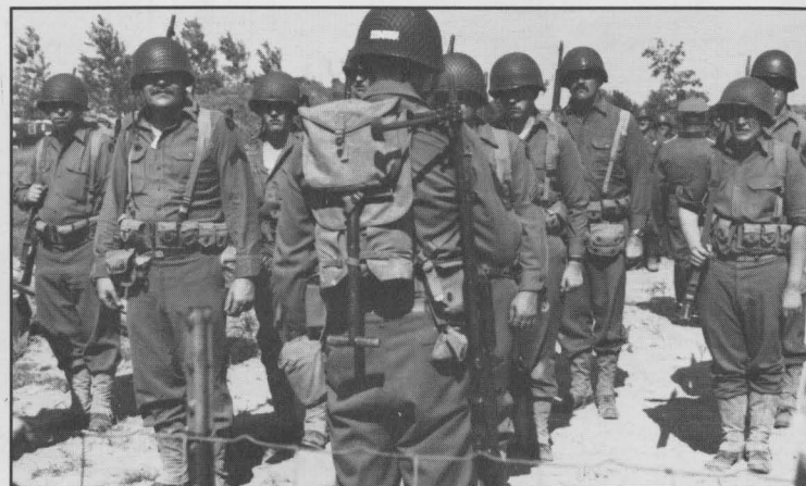
Memorial Day Weekend 1985, "ready for inspection"
